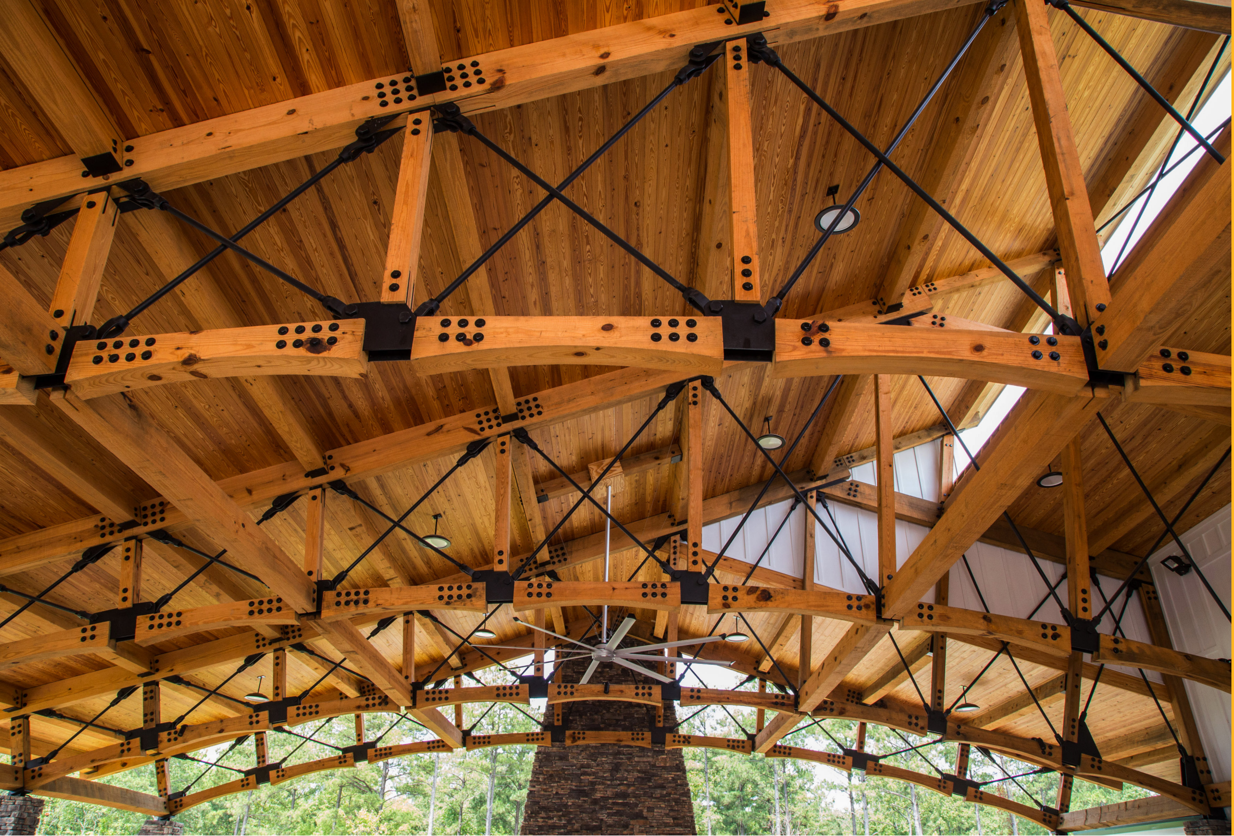
NWTF Palmetto Shooting Complex Pavilion and Education Center
