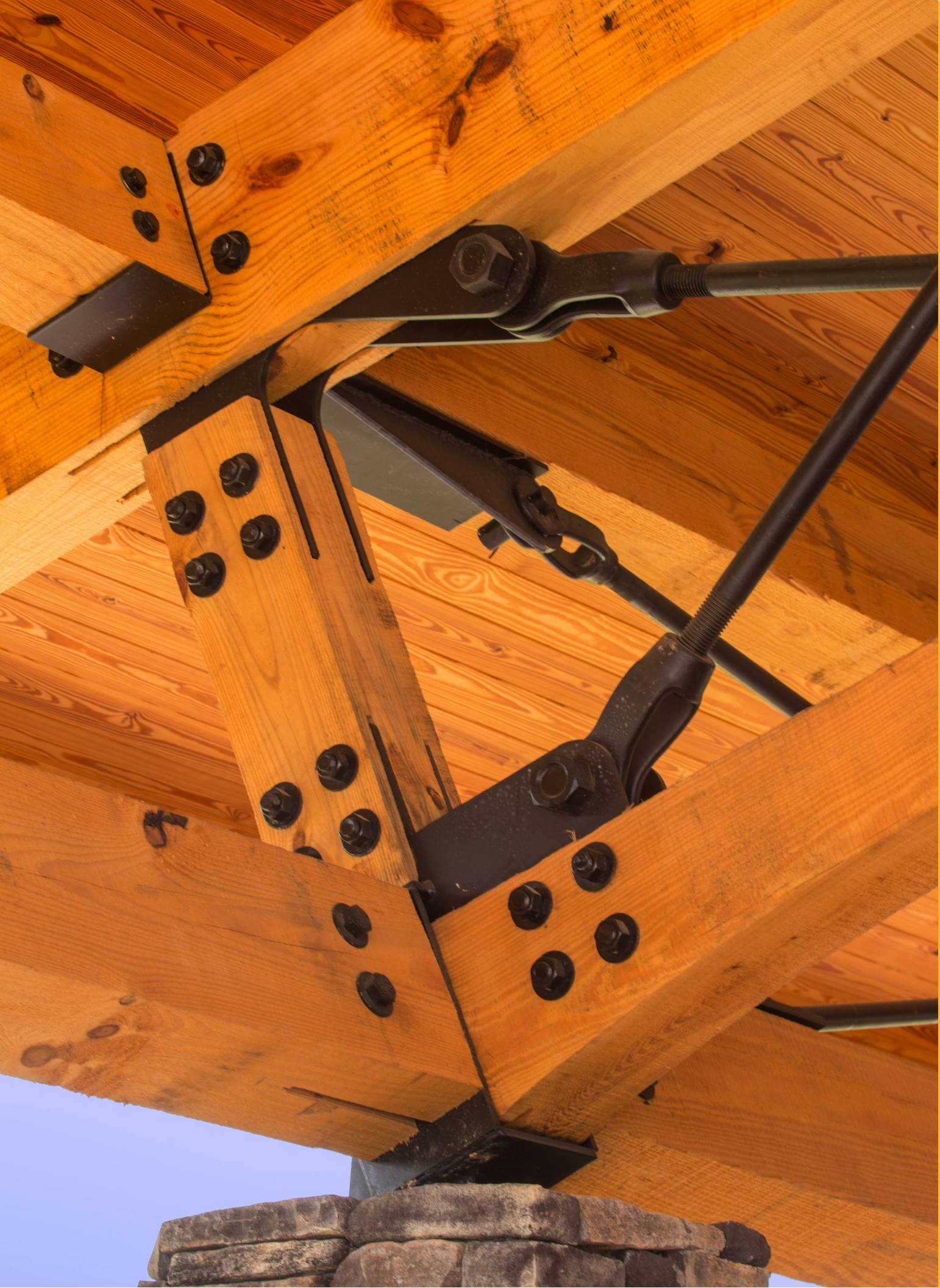
NWTF Palmetto Shooting Complex Pavilion and Education Center
